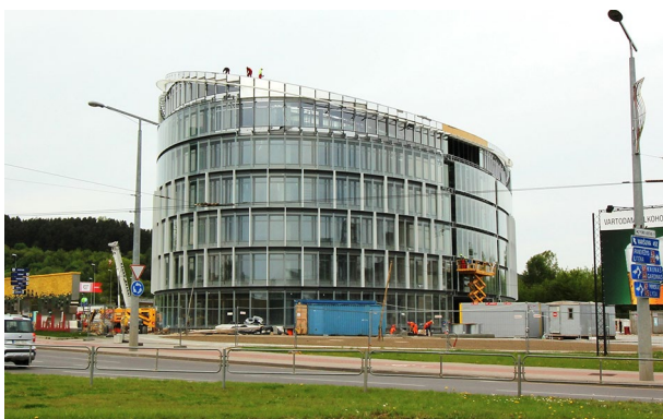
Fig. 1. An original office building, Vilnius
