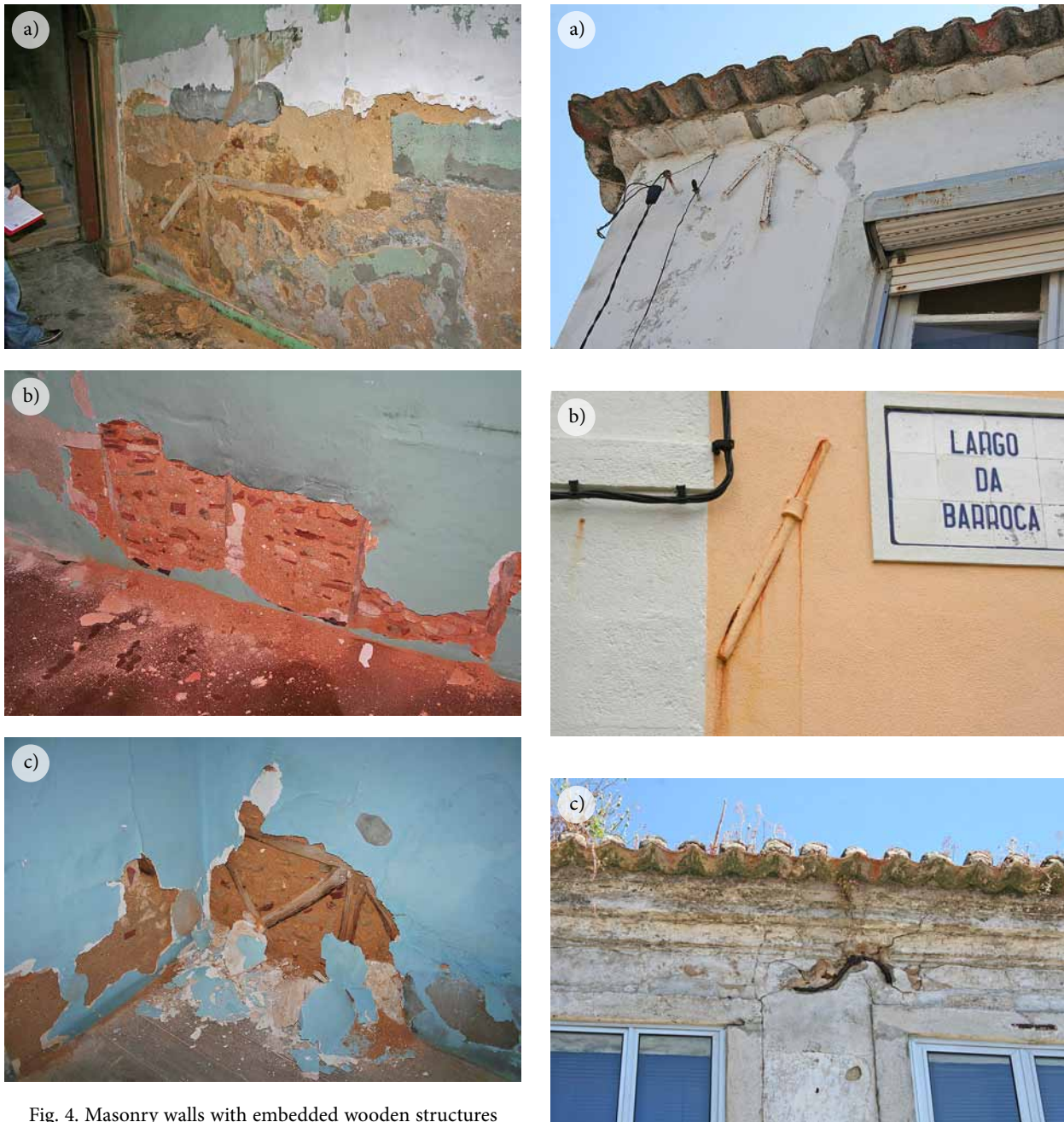
Fig. 4. Masonry walls with embedded wooden structures
