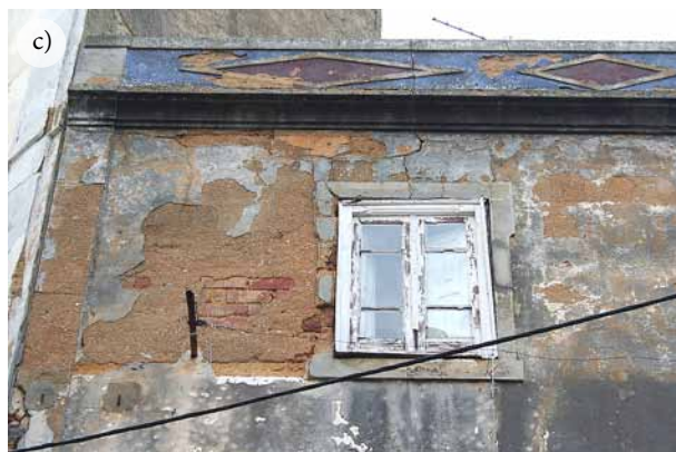
Fig. 3. External aspect of some of the most common masonry types
