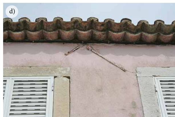
Fig. 5. Examples of tie rods observed in the old centre of Seixal
