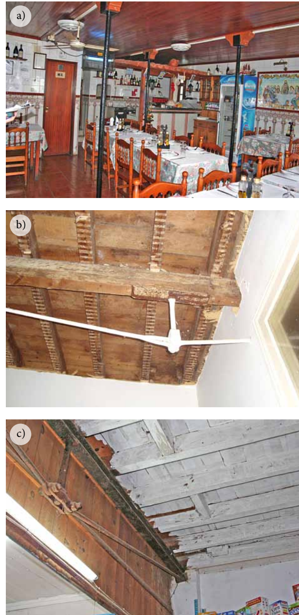
Fig. 8. Original constructive solutions strengthened with metallic elements
