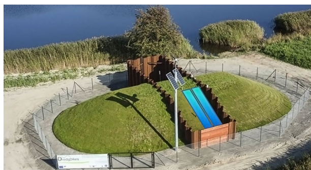
Fig. 3. Gdansk research dike with test section and location of flume 1 (right) and flume 2 (left)
