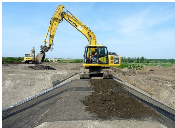
Fig. 14. Installation of the erosion control product
