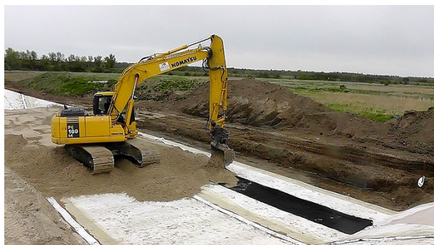
Fig. 12. Installation of the geosynthetic clay liner and drainage composite
