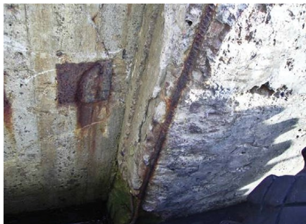
Fig. 10. Valve lesions at the quay of the Port of Klaipeda
