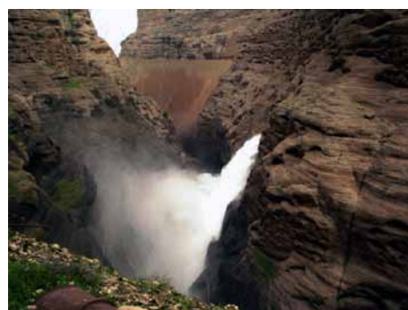
Fig. 5. Deep valleys with low width in the Dez Dam
