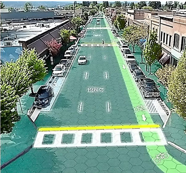
Figure 1. Hexagonal Solar Panels with toughened glass installed on road surface (Solar Roadways Incorporated, 2020)
